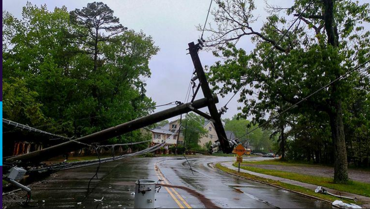
Road Debris Clearance Cut & Push | Reopen
